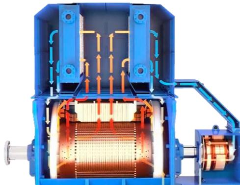
Figure 2. Turbogenerator cooling system.
